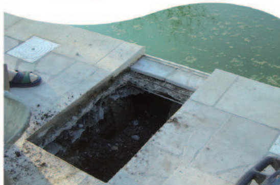
6 - End of large work
